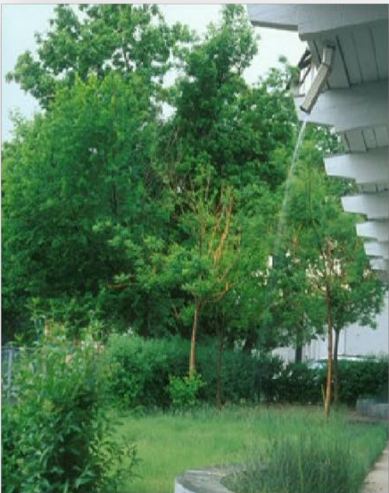
Irrigation by disconnected downspout Denver, CO
