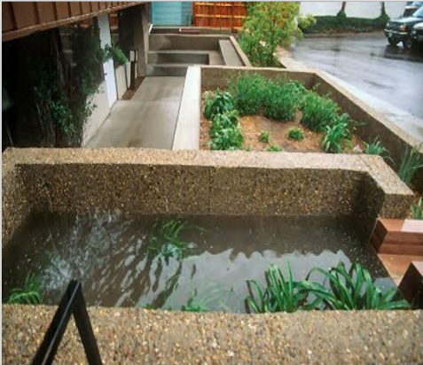
Rainwater collected in planter box then channeled into rain garden Boulder, CO
